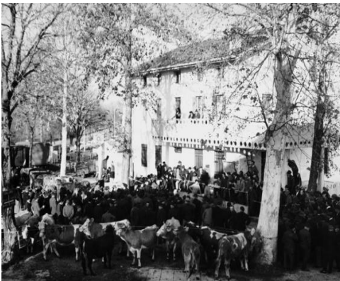
Figure 24 Historical picture of the Delle Acque Place
